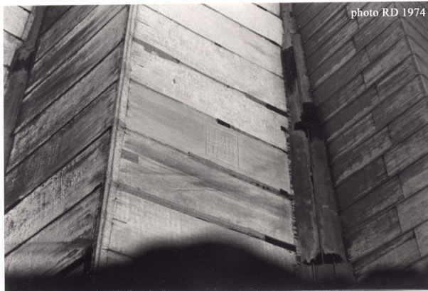
THE LEAD ROOFS OF 1829
