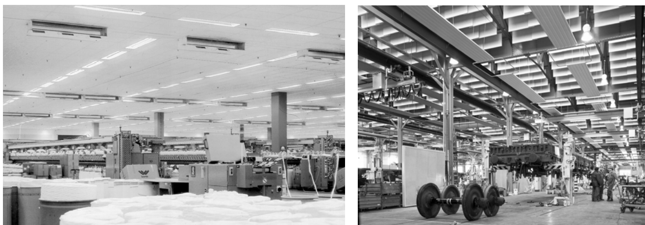
Fig. 4.4.2 Examples of acoustic treatment mounted in ceiling in industrial halls. Left: suspended ceiling of mineral wool tiles with integrated light fixtures. Right: Vertical Mineral wool baffles.
