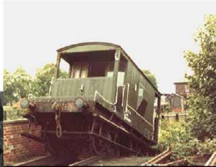
Rail collapse leads to derailment of a locomotive in Driffield, UK, in 1981
