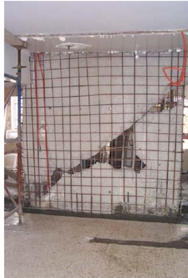
Photo 03: Steel reinforcement
